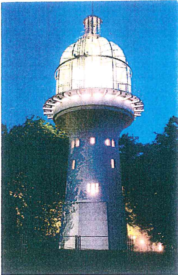
old water tower in Solingen (Germany) converted into a light tower as a conference room with glass dome
